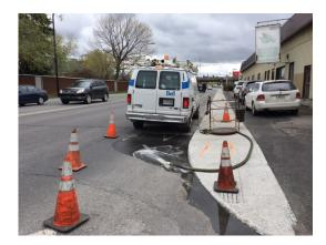
Adherence to this procedure seeks to ensure that contaminated effluent is identified before the manhole is pumped, thereby protecting surrounding land and water bodies from these contaminants.
