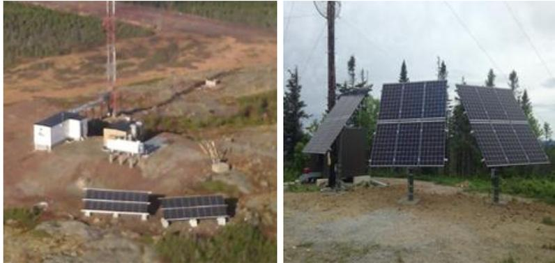
In 2022, Bell Mobility will also complete coverage of Highway 6 in Manitoba with the addition of two new off-grid sites. These sites will be equipped with the latest iteration of high efficiency photovoltaic solar panels, made for cyclic use lithium batteries, DC fan cooling and DC Generators, and almost all shelter components will be DC powered.
