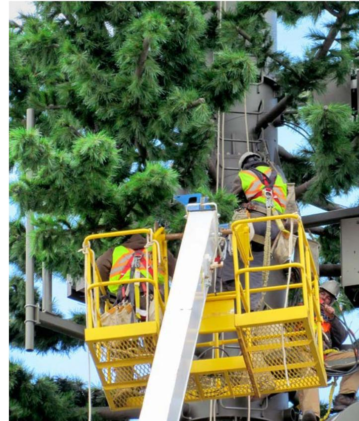
First and Only Canadian designed pine tree in Milford Bay (Muskoka), Ontario. One week was required to complete the build. In this picture the rigging crews are making the final connections between the radios and the antennas.
