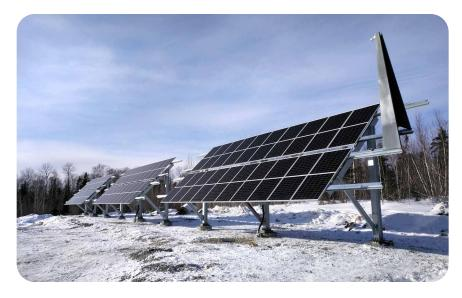
A 2021 research project, a collaboration between Bell, Québec-based solar energy company Stace and Université de Sherbrooke, studied the viability of these solar voltaic cells to generate renewable energy to provide primary power for remote telecommunications towers – displacing diesel generators and reducing the associated greenhouse gas emissions.
